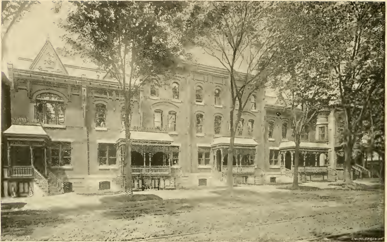
ROW OF BRICK RESIDENCES, PENNSYLVANIA AVENUE, NEWARK. BUILT BY CONRAD, WOOD & HELLINGS OF PHILADELPHIA, PA.
